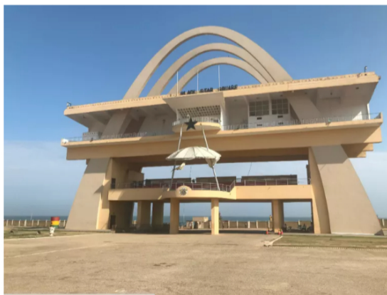
Ghana Independence Arch, Accra by Public Works Department built by Kwame Nkrumah for Queen Elizabeth's visit to Ghana in 1961 (Image credit: Victoria and Albert Museum, London)
