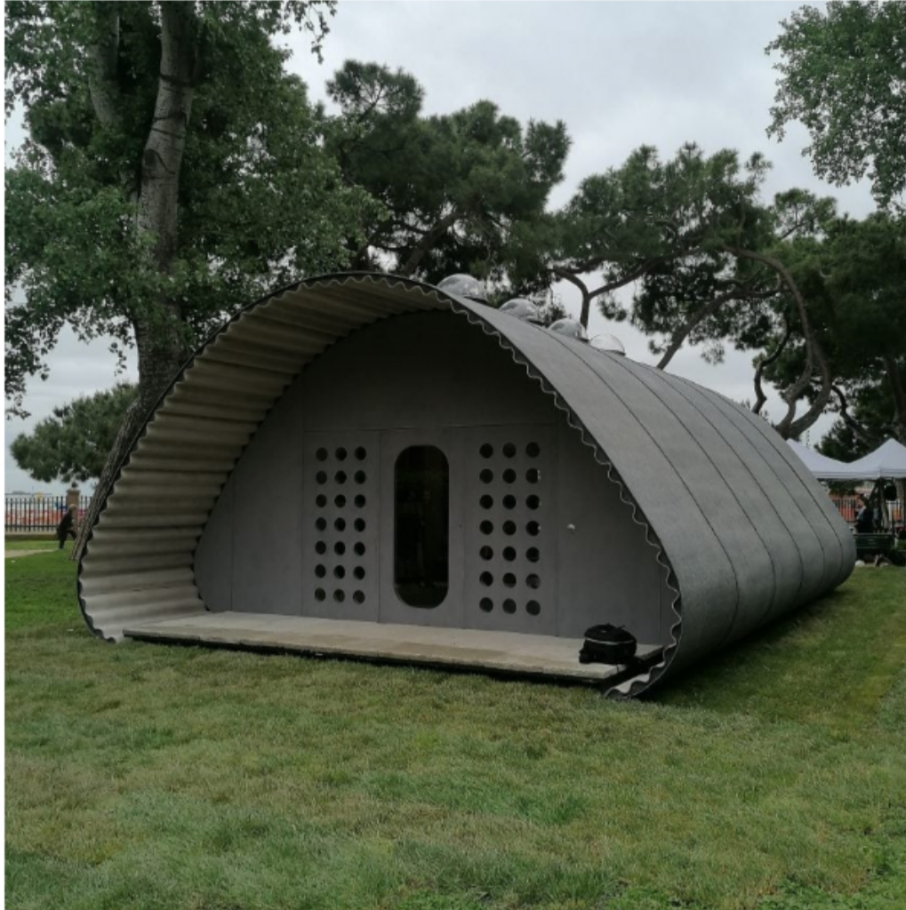
The Essential Homes Research Project is a concept designed to sustainably provide rapidly assembled housing for people displaced by natural and manmade disasters.
